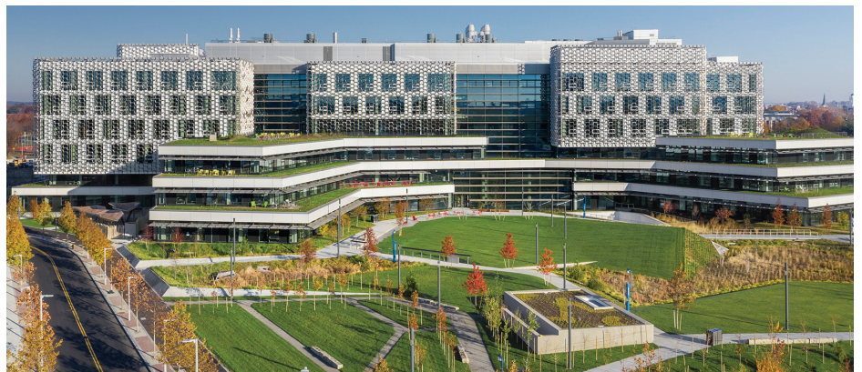
Home to the Harvard John A. Paulson School of Engineering and Applied Sciences (SEAS), the 544,000-sf building is a living laboratory for interdisciplinary research, learning, and innovation.
